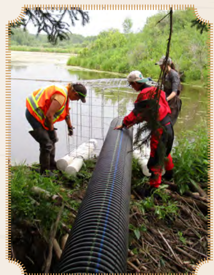
Installing a pond leveller. GLYNNIS HOOD
