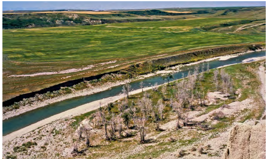
Top: The depleted Oldman Reservoir after drought conditions in 2001. Droughts of more than two years in duration cannot be mitigated with reservoir storage. The irrigation sector needs to factor climate change into any expansion plan. LORNE FITCH
